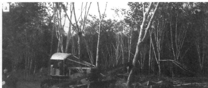
(a) Uprooting by bulldozer
