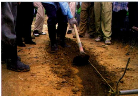
(a) Preparing trenches for polybag buddings
